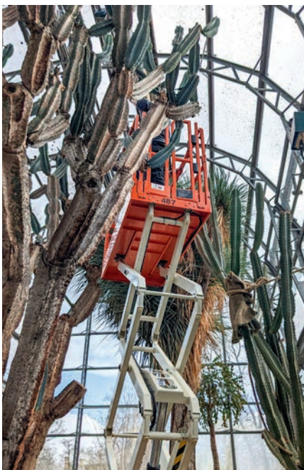
Repairing the Arid House
